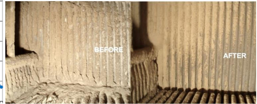
A region of the superheater before and after the installation of the SMART Helix Water Sootblower
